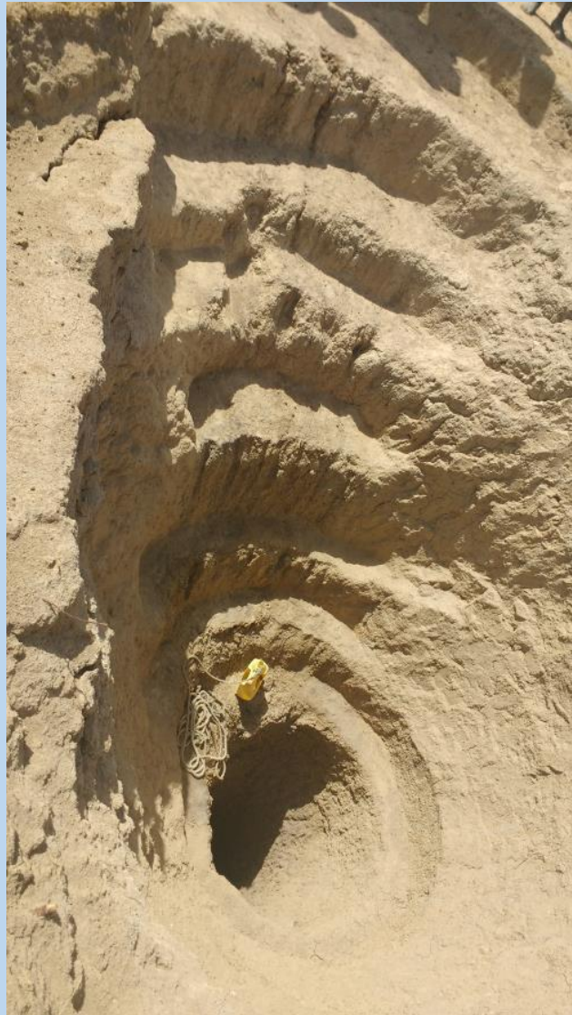
Hand-dug shallow well, low water table
