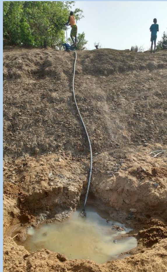
Hand dug well in dry river bed with treadle pump
